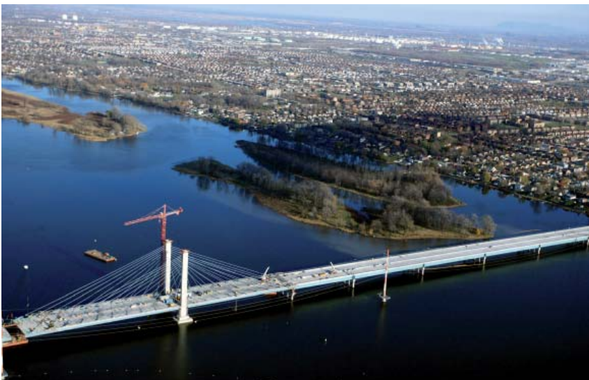
Aerial view of autoroute 25's bridge under construction
